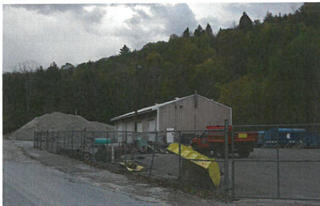
The highway garage also is the site of the Town's transfer station.
