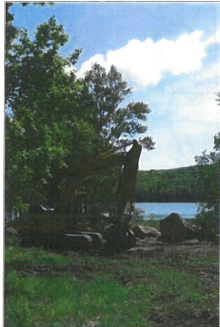
Recent work at the shore of Sucker Pond reduced erosion and improved water quality and public access (US Forest Service photo).
