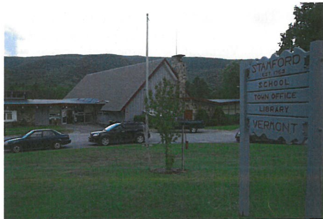
The Stamford School is an important community resource.
